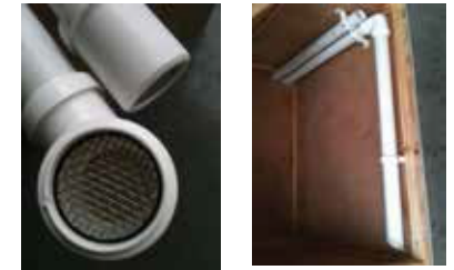
Dip and vent tubes exit through side of hut to exterior Hydrogen gas vet tube turns up at end, cold air tube is a straight exit. Both tubes have mesh covering to prevent insects from entering
